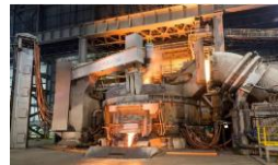
Electrical arc furnace
